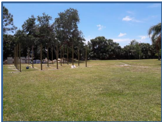
Figure 19. Above shows the construction site of the future Satellite Beach community garden.
