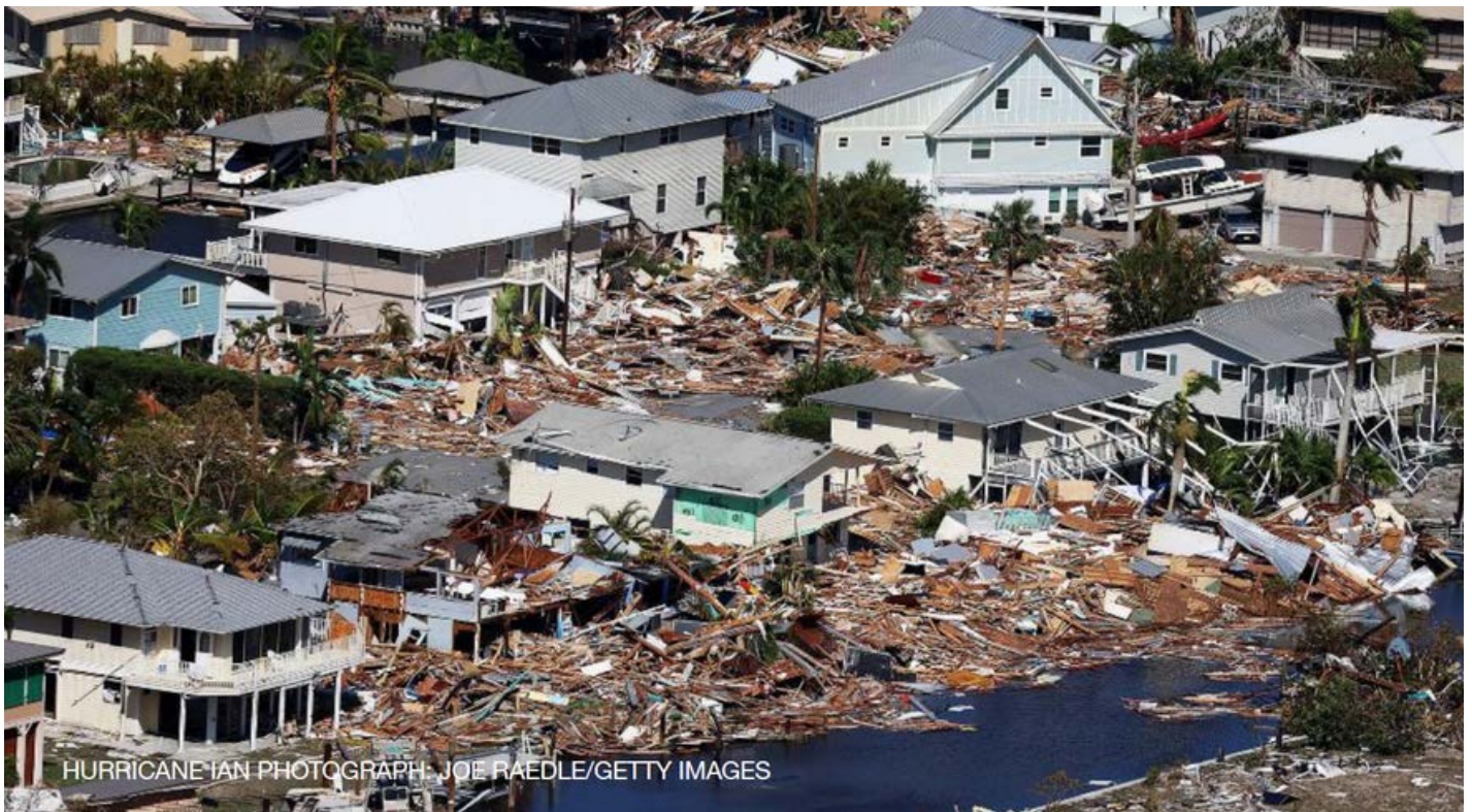
Photo of Hurricane Ian damage in 2022 on west coast of Florida, credit: Joe Raedle
