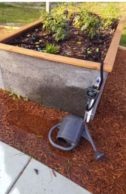
Photo of a leaking hose at garden, credit: Thea Baker
