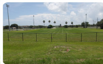
New Fencing 715 Linear Feet
